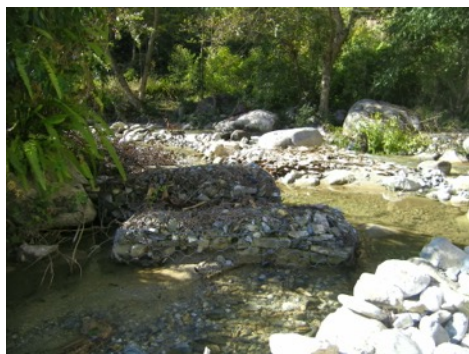
Gabions to divert water to an intake tank
