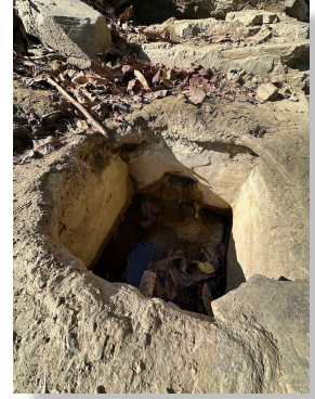
Buried water tank
